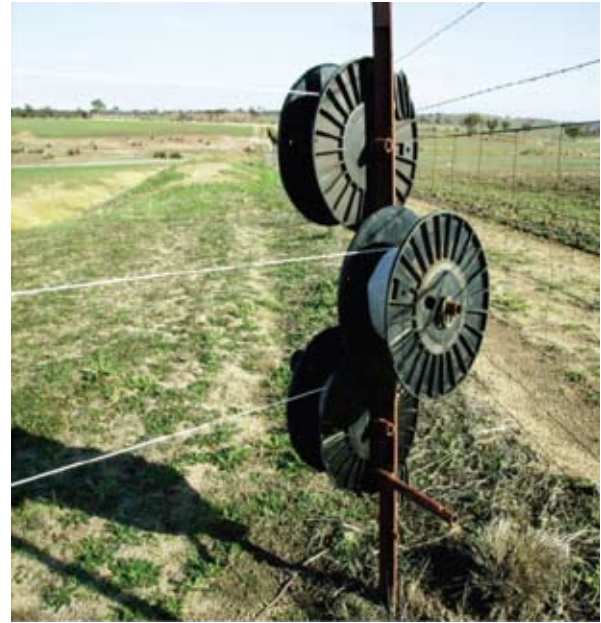
Installing temporary fences with a Rappa Fence Systems™
